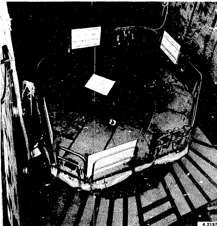
Figure 26. IIF installed on reactor vessel flange.
